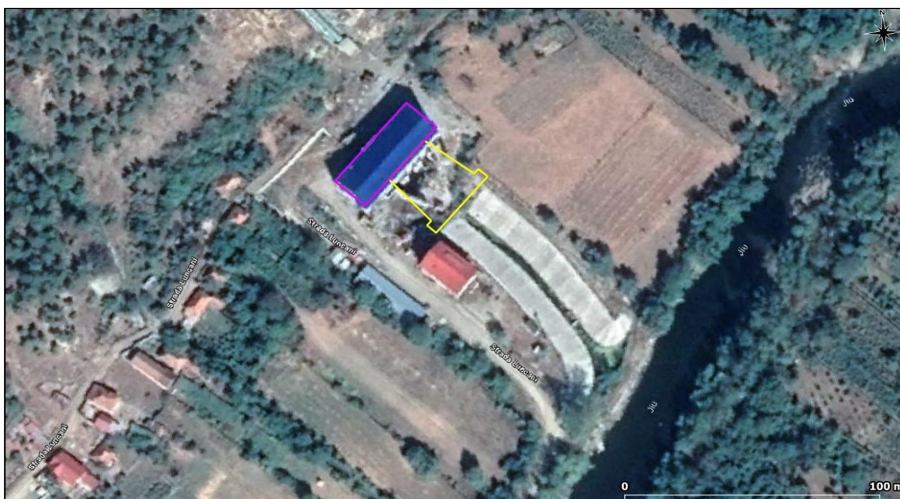
Fig. 37 The territorial framing of the CHE Bumbești building (purple polygon) and of the connection area between the CHE Bumbești stilling basin and the escape channel (yellow polygon)
