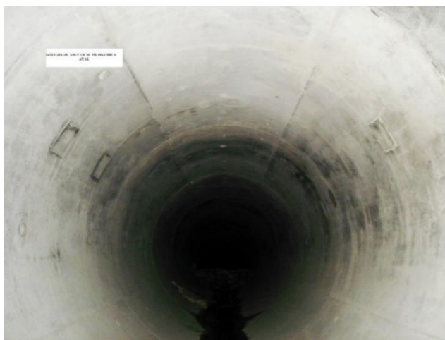
Fig. 16 Concrete intake Murga downstream
