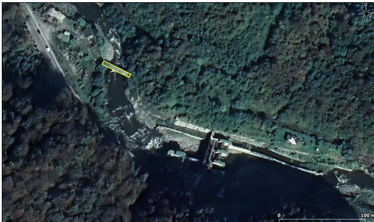
Fig. 43 Spatial delineation of the temporary bridge upstream of the Livezeni dam (yellow polygon)
