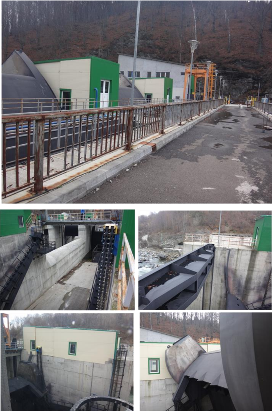
Fig. 9 Physical status of the Livezeni Dam
