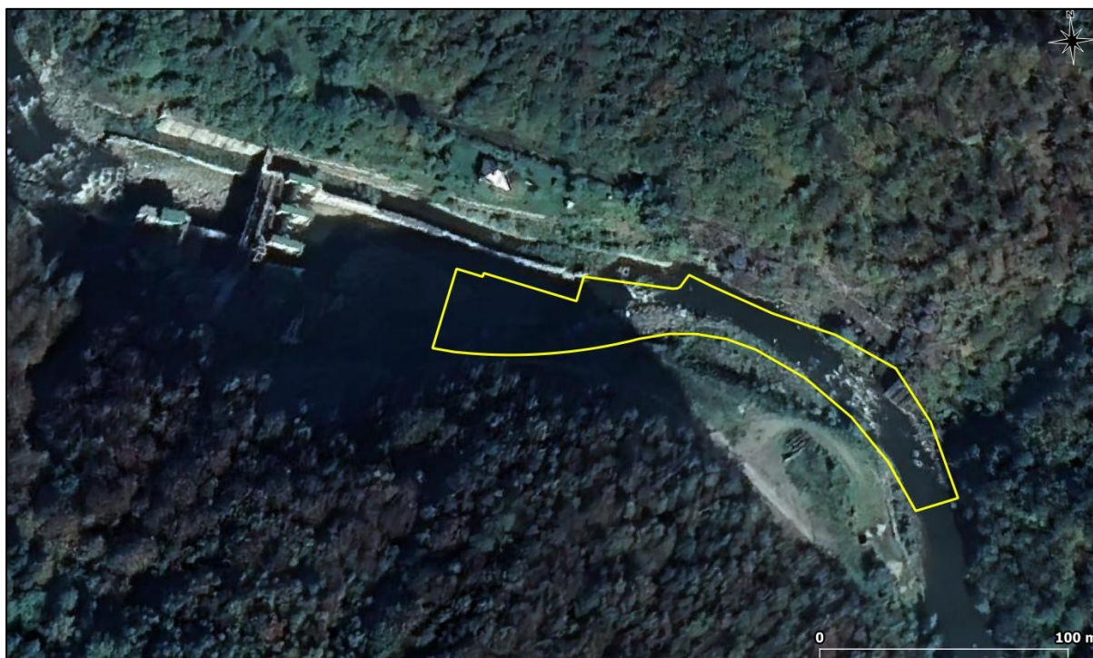
Fig. 29 Location of the section of the Jiu riverbed targeted by regularization works downstream of Livezeni dam
