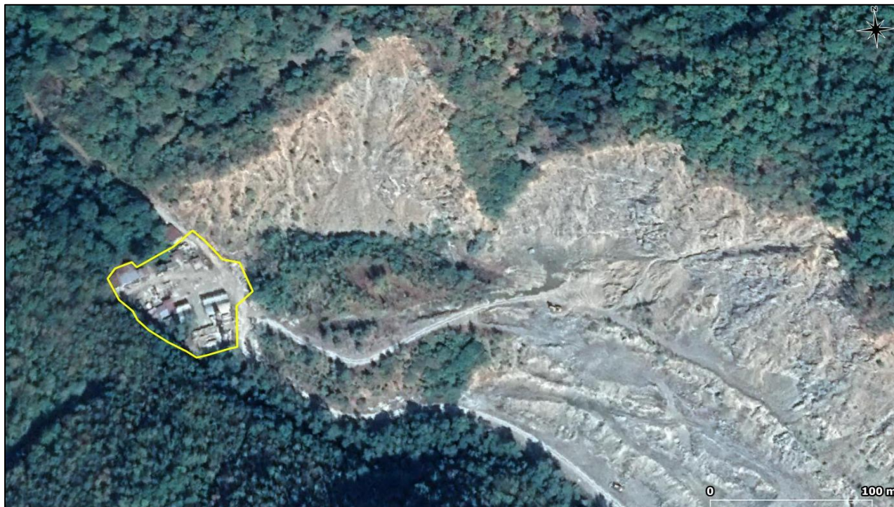
Fig. 47 Territorial framing of the site organization at the Bratcu Tunnel (yellow polygon), target of decommissioning works
