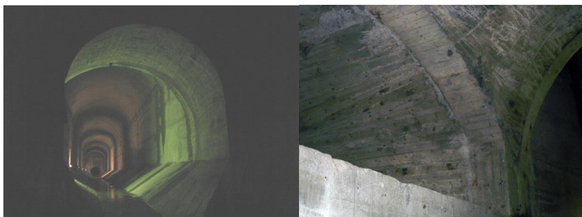
Fig. 17 Pictures inside the concrete settling tank
