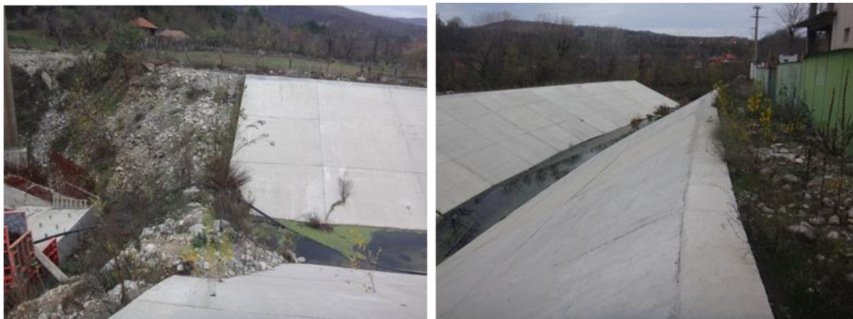
Fig. 20 Flume at the connection to the stilling basin and long view
