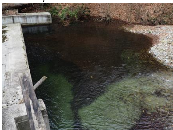
Spillway dam area
