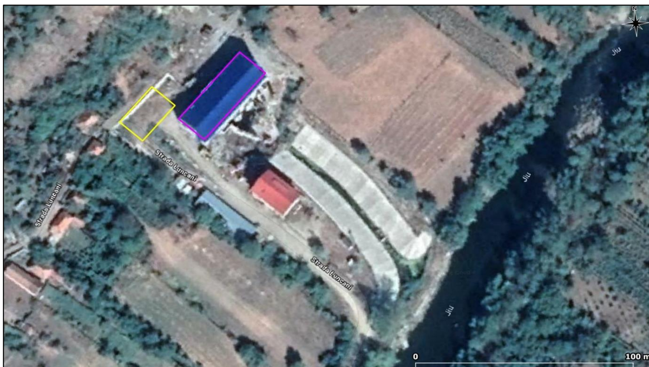
Fig. 38 Territorial framing of the CHE Bumbesti building (purple polygon) and the 110 kV CHE Bumbesti transformer station (yellow polygon)
