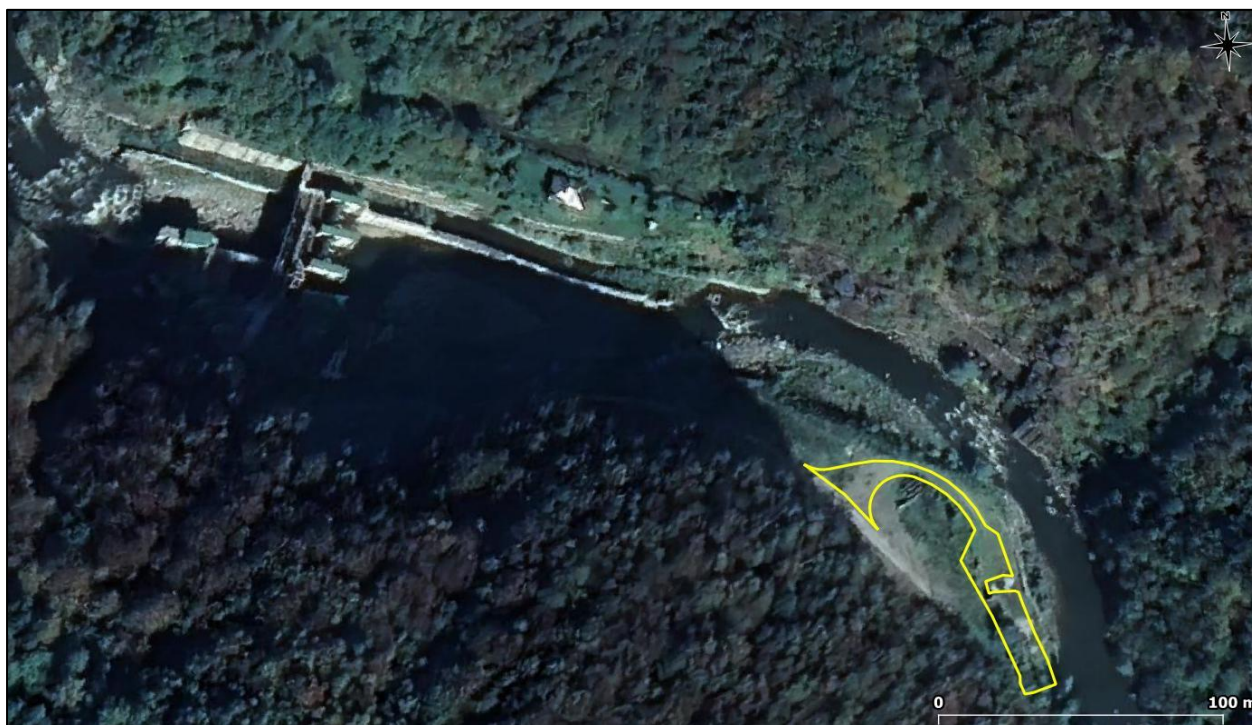
Fig. 45 Spatial setting of the technological platform and the access road to the Livezeni access tunnel (yellow polygon), objectives targeted by the development works
