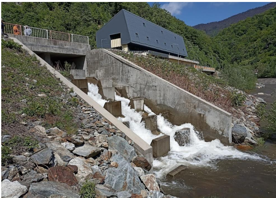
Fig. 181 Image of the interruption of longitudinal connectivity at the level of the confluence of the Dumitra stream with the Jiu River
