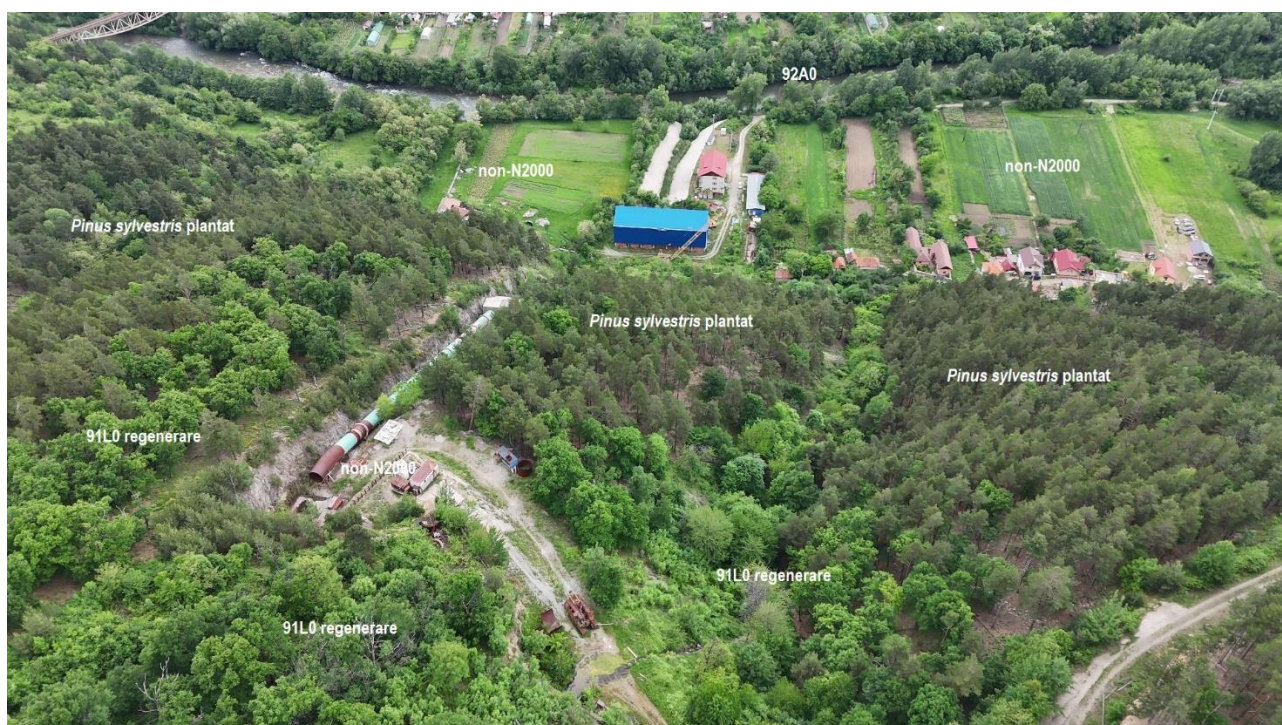
Fig. 91 Detail of the N2000 and non-N2000 habitats of the southern mountain range, in which the CHE Bumbesti is embedded, the area of the penstock
