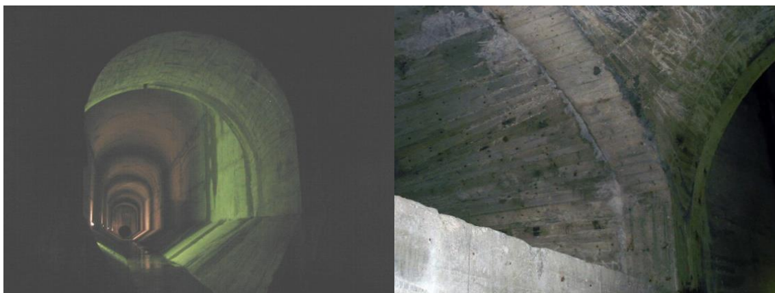
Fig. 12 Pictures inside the concrete settling tank
