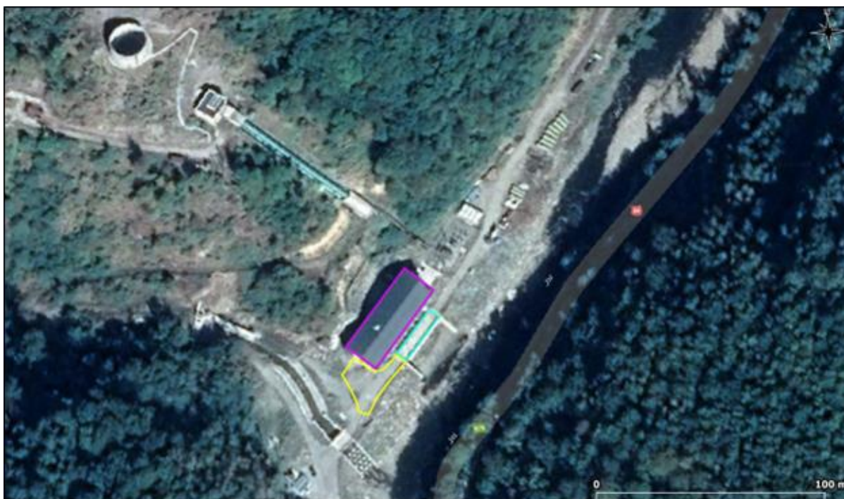
Fig. 30 Territorial framing of the CHE Dumitra building (purple polygon), the Dumitra power plant platform (yellow polygon) and the bridge over the stilling basin (blue polygon)
