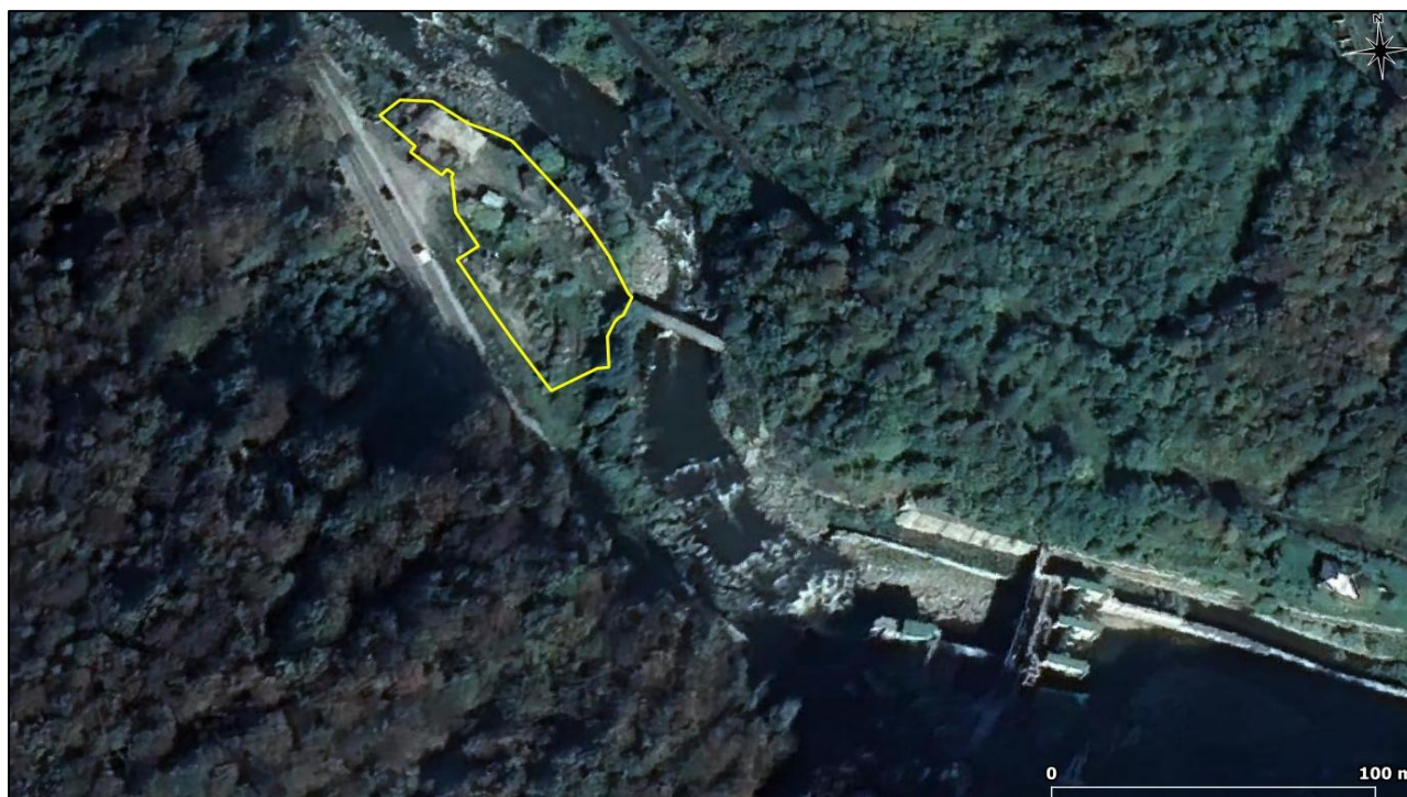
Fig. 44 Spatial delineation of the technological platform located upstream of the Livezeni dam (yellow polygon), targeted by decommissioning works
