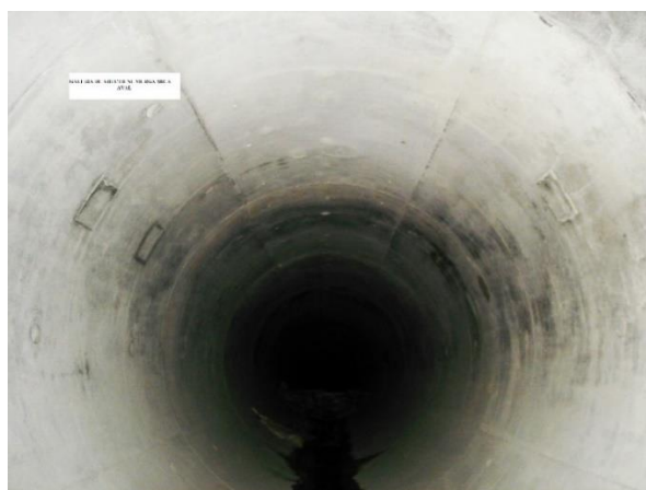
Fig. 11 Concrete intake Murga downstream
